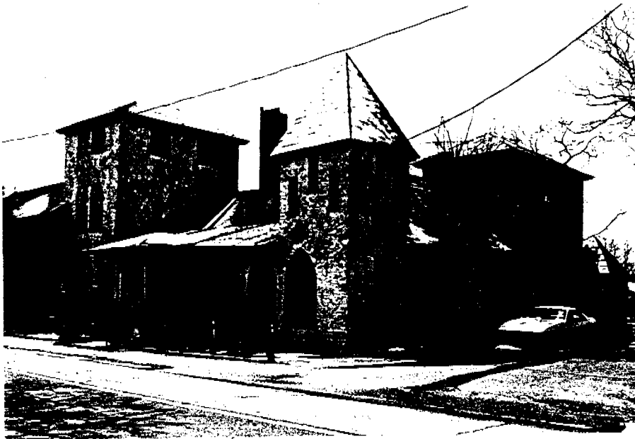
Neg. KK XIX-10, fm. NE, view of Smithtown Avenue facade.
