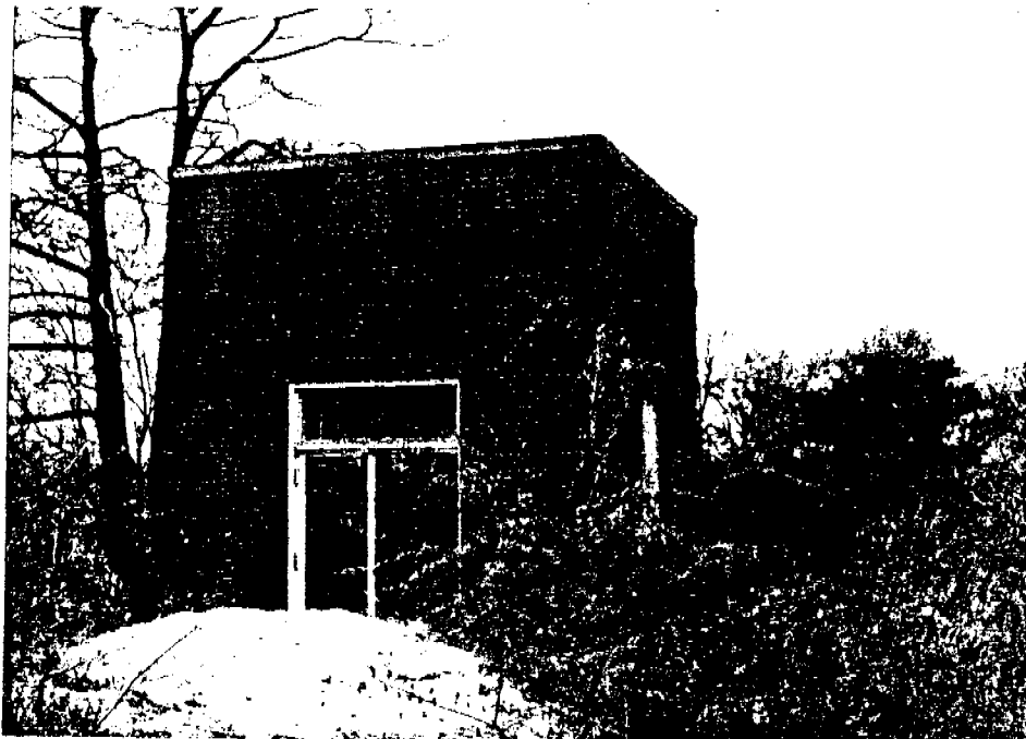
BUILT C 1940, BLDG. 131, RED BRICK
