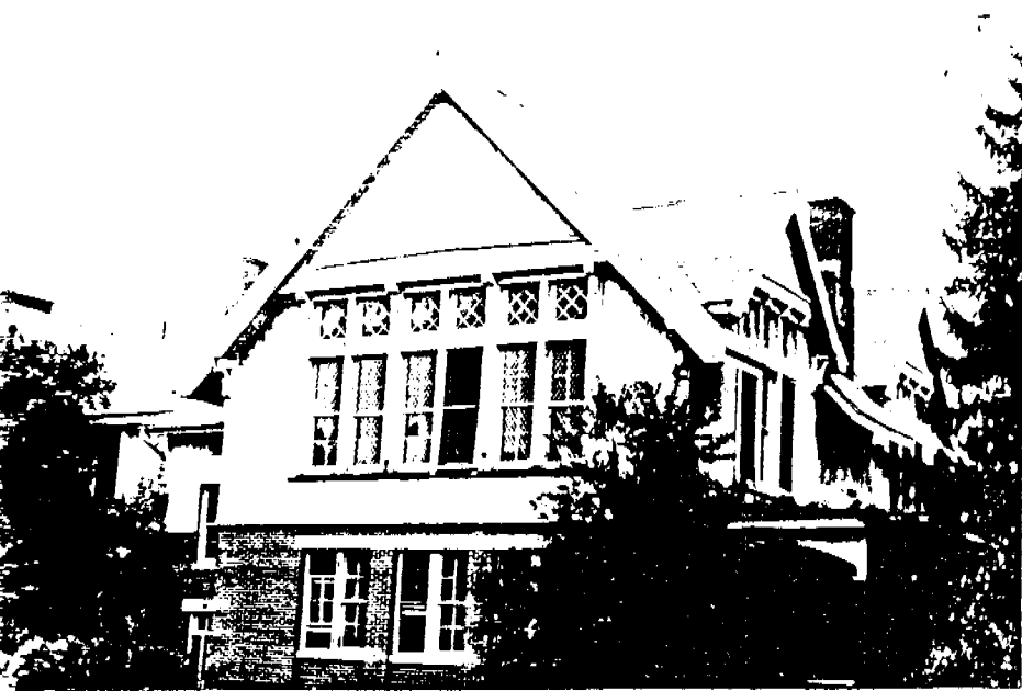
Roll #Q7; Neg. #2 HP-1 Building in M Group
