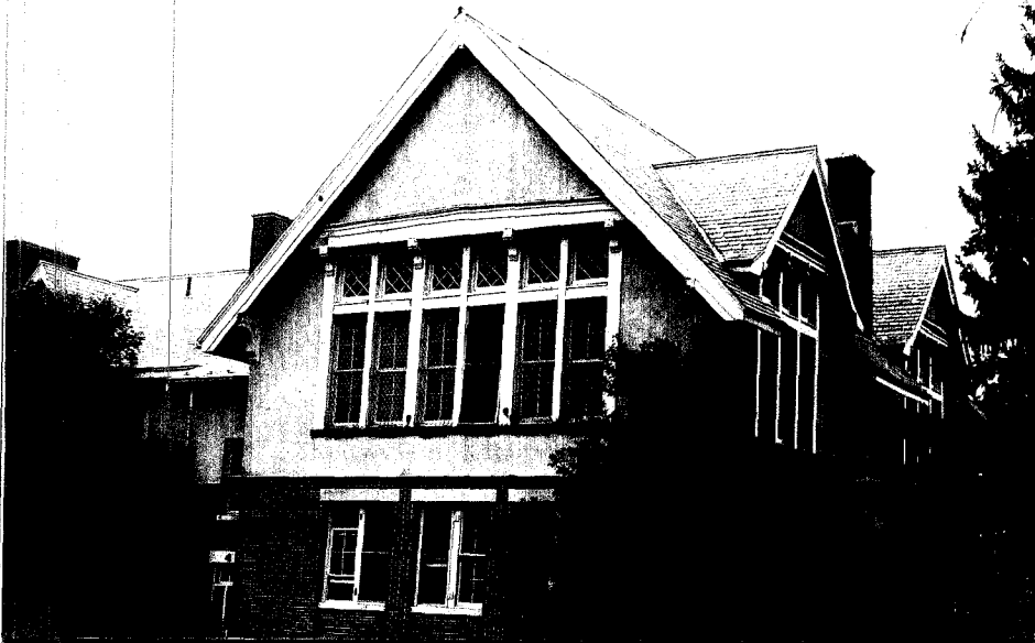
HP-1 Roll #Q7; Neg. #2 Building in M Group
