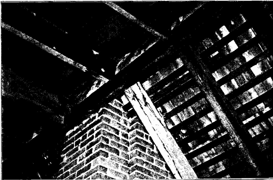
Photograph 26 – Staining of the roof framing indicates long-term leaks around the chimney.
