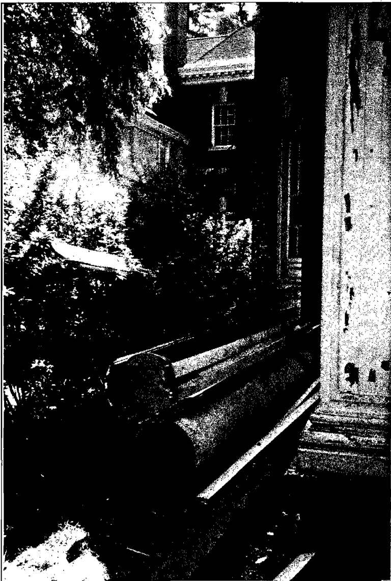
Photograph 56 – Original columns removed from the west portico are rotting away in the nearby bushes.
