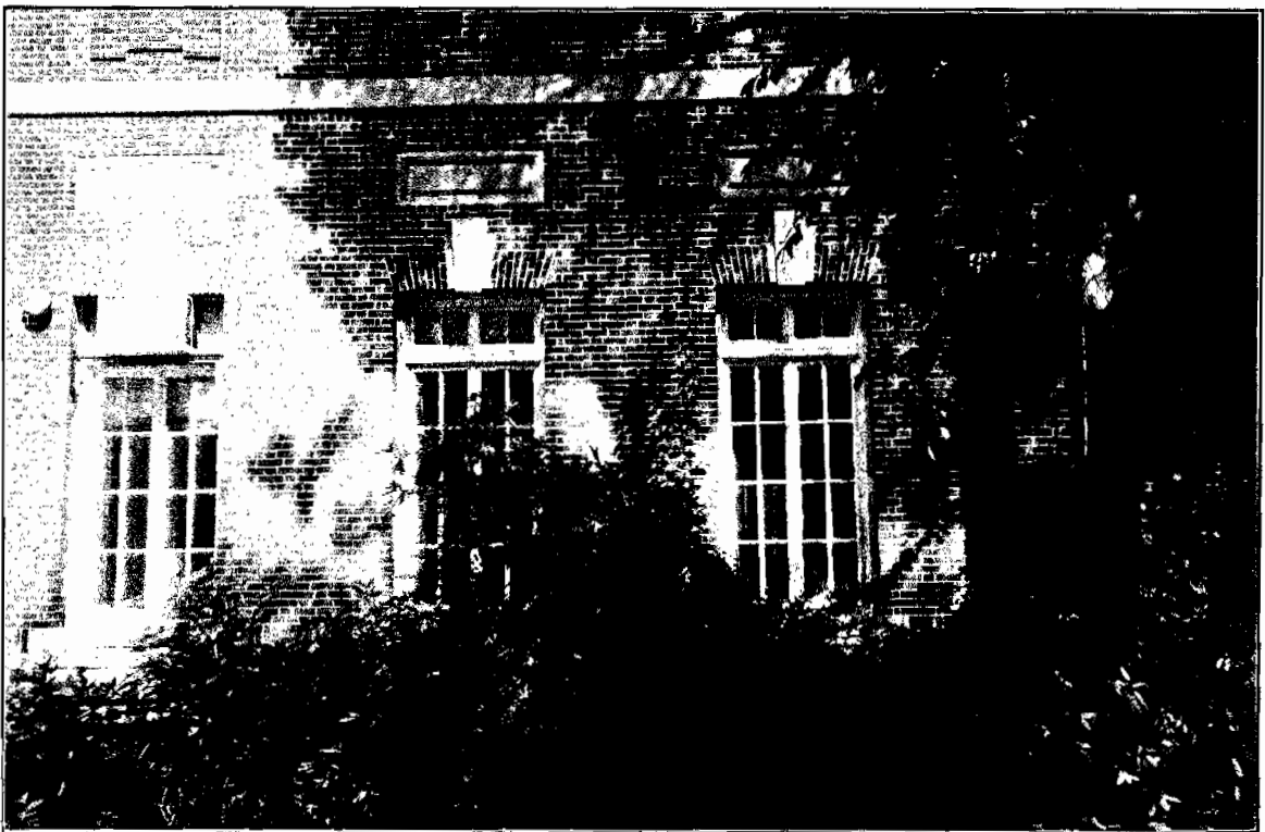
Photograph 42 – The low landscaping and creeper climbing the building both keep moisture against the masonry, accelerating deterioration of both brick and mortar.
