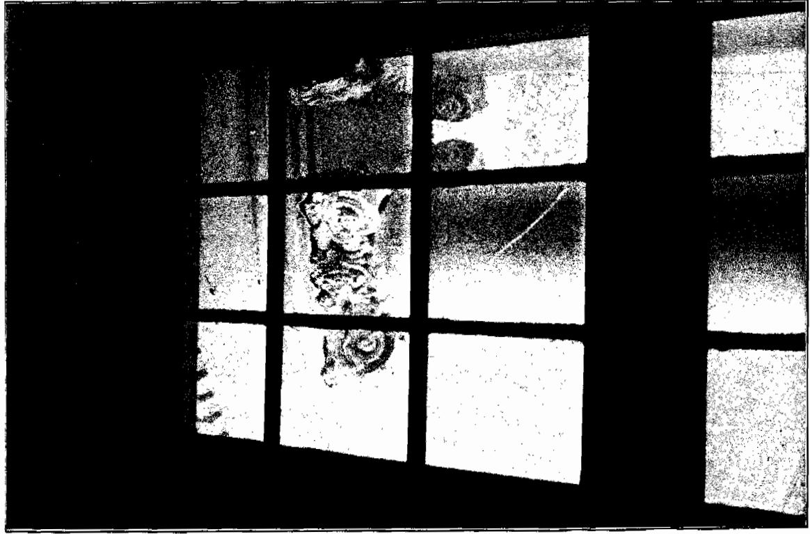
Photograph 9 - Cracked and broken panes of glass should be repaired promptly, using matching glass, not Plexiglas.
