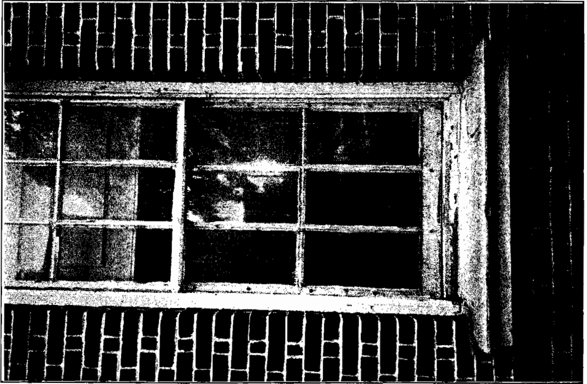
Photograph 49 - Plexiglas has been affixed directly to this window sash.
