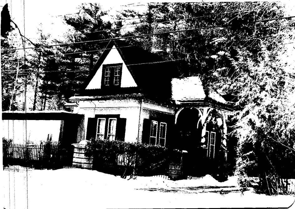
HP-1 Looking southwest
