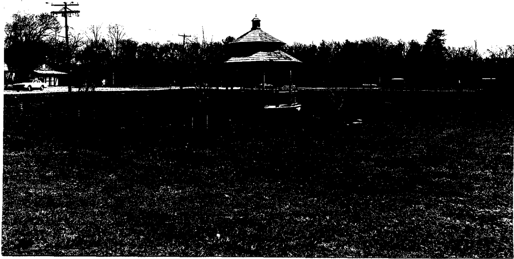
Neg. KK XXII-30, fm. N. Gazebo constructed on the site in 1987.
