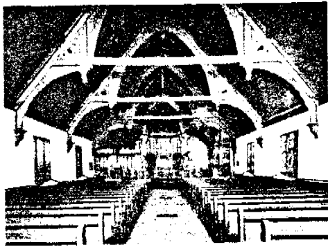
37. ST. MARK'S EPISCOPAL CHURCH, ISLIP Richard Morris Hunt, Architect 1878-80
